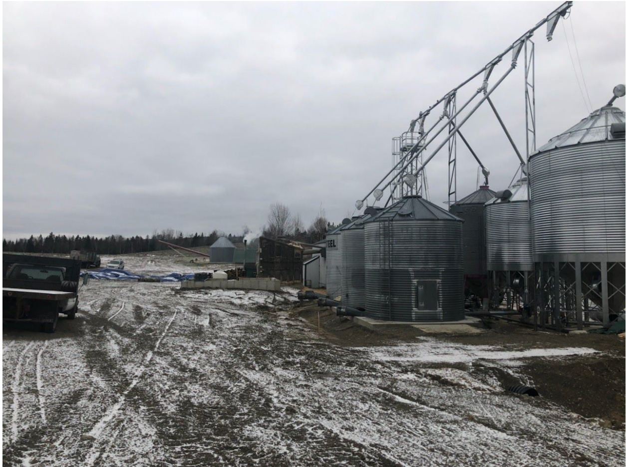
Another view showing the looping system at Aurora connecting to the mill and cleaning systems.
